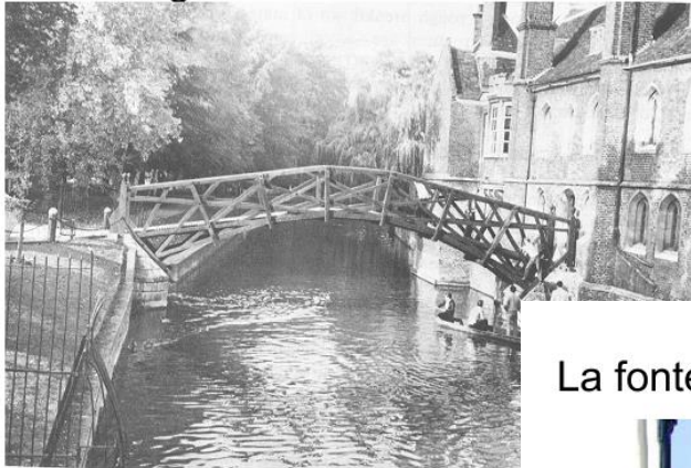
Le bois, reconstruction 1904 original 1749
