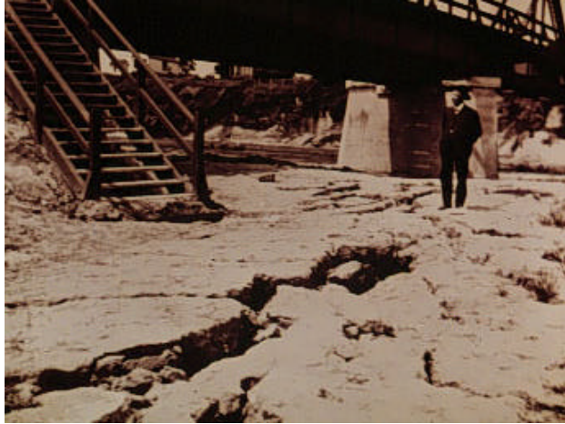
Fig. 6.8(a) Crack formation due to liquefaction (Courtesy: http://www.es.ucsc.edu )
