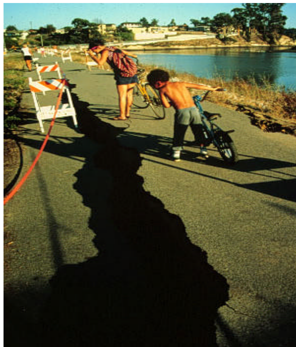
Fig. 6.7 Failed river dike due to liquefaction (Courtesy: http://www.es.ucsc.edu )
