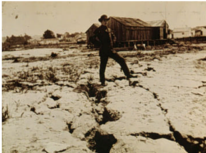
Fig. 6.8(b) Crack formation due to liquefaction (Courtesy: http://www.es.ucsc.edu )
