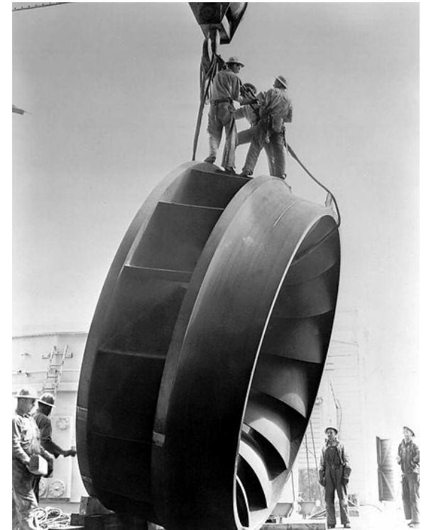
Francis Runner, Grand Coulee Dam
