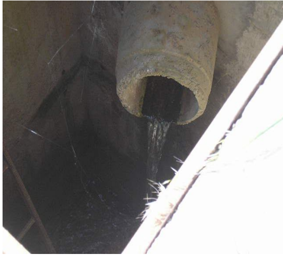
Figure III.38. Drainage de la source N° 01, rive gauche, barrage Sikkak, wilya Tlemcen [70].
