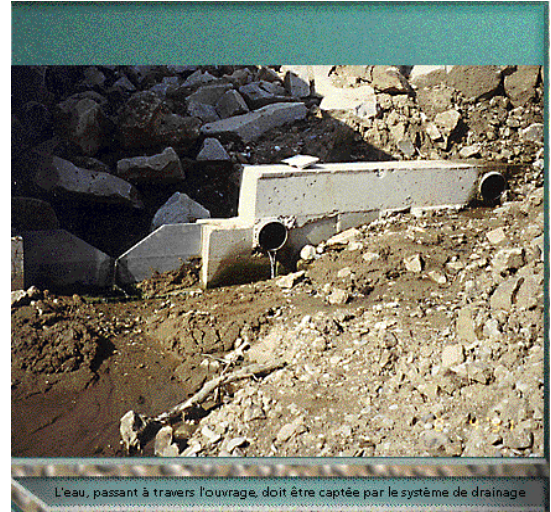
Figure III.38. Drainage de la source N° 01, rive gauche, barrage Sikkak, wilya Tlemcen [70].
