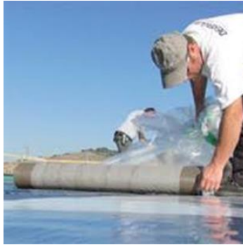
Figure 26 : La membrane derbipure
