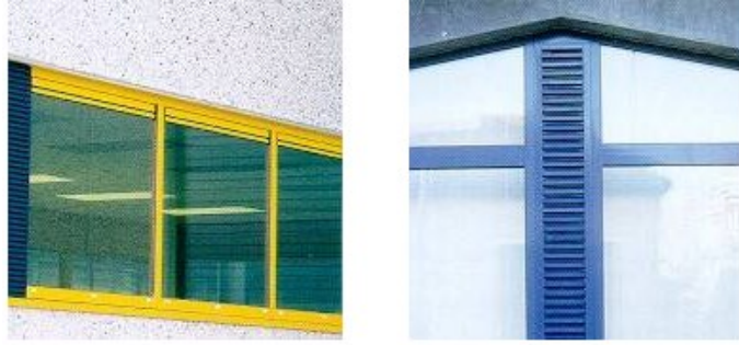
Figure 44. Grilles de ventilation
