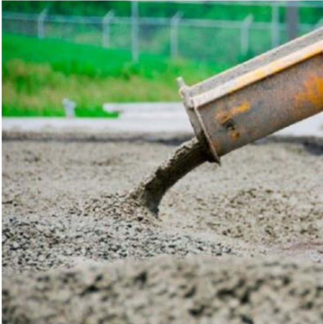
Ready-mixed concrete liquefied with a plasticiser
