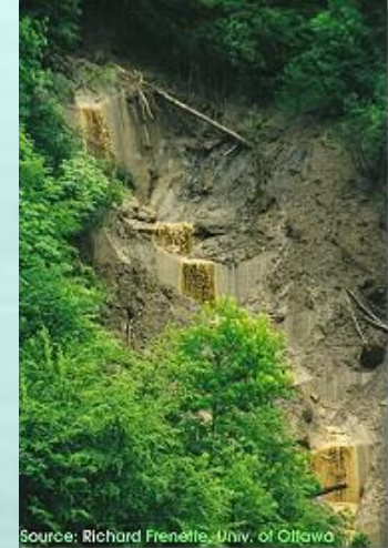
Landslide from heavy rainfall – needs protective measures
