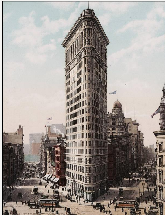
Flatiron Building (87 m) New York (1903).
