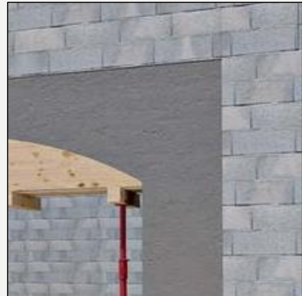
Reinforced Concrete Springer
