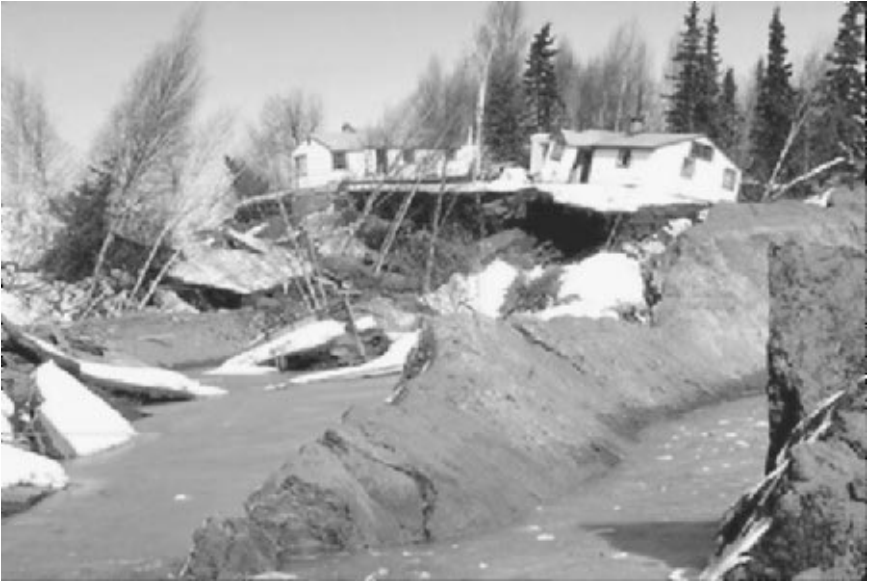
FIGURE 3.51 Damage caused by movement of the Turnagain Heights landslide during the Prince William Sound earthquake in Alaska on March 27, 1964. (Photograph from the Steinbrugge Collection, EERC, University of California, Berkeley.)
