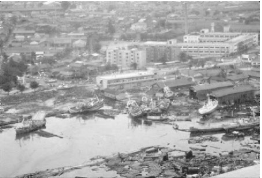
FIGURE 3.56 Tsunami damage caused by the Niigata earthquake in Japan on June 16, 1964. (Photograph from the Steinbrugge Collection, EERC, University of California, Berkeley.)
