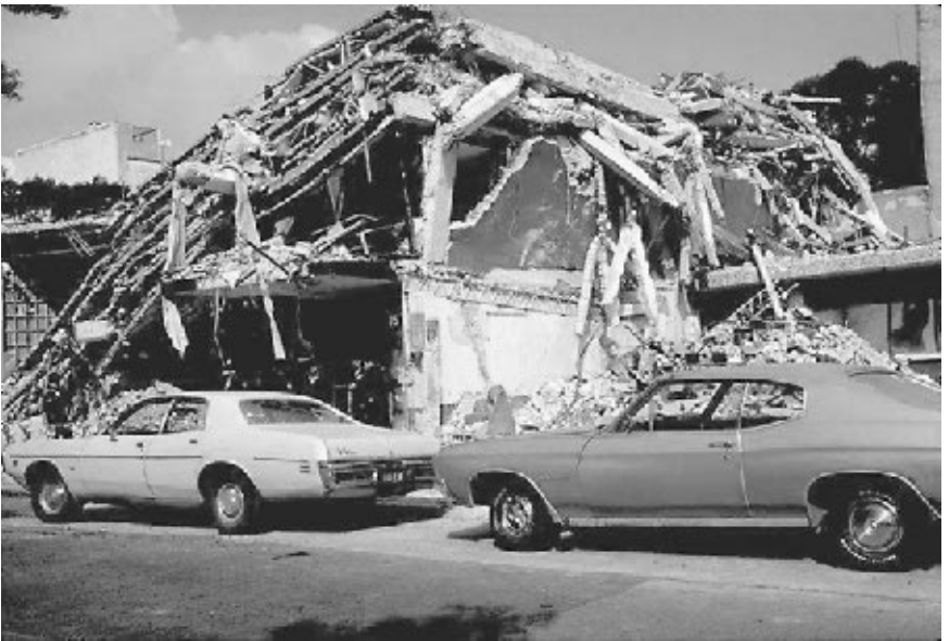
FIGURE 4.24 Building collapse in Mexico City caused by the Michoacan earthquake in Mexico on September 19, 1985. (Photograph from the Steinbrugge Collection, EERC, University of California, Berkeley.)
