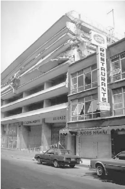
FIGURE 4.17 Pancaking of the upper floors of a parking garage during the Michoacan earthquake in Mexico on September 19, 1985. Note that the restaurant building provided additional lateral support which enabled the lower three floors of the parking garage to resist the collapse. (Photograph from the Steinbrugge Collection, EERC, University of California, Berkeley.)
