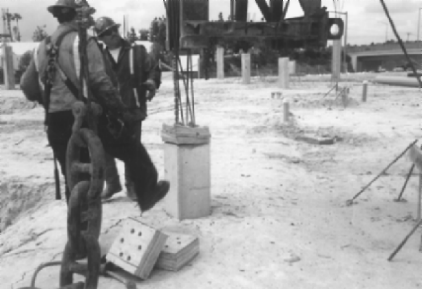
FIGURE 13.21 A prestressed concrete pile has been successfully driven to the bearing strata. The wood block shown on top of the concrete pile was used as a cushion to protect the pile top from being crushed during the driving operation.
