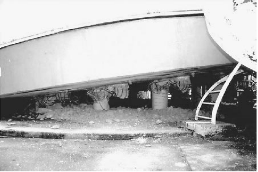
FIGURE 4.12 Overview of a collapsed gas storage tank, located at a gas storage facility near Sabanci Industrial Park, Turkey. The elevated gas storage tank collapsed during the Izmit earthquake in Turkey on August 17, 1999. (Photograph from the Izmit Collection, EERC, University of California, Berkeley.)
