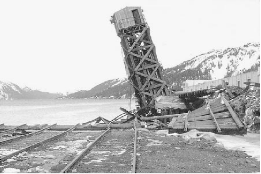
FIGURE 4.2 Close-up view of the tilted tower shown in Fig. 4.1. The tilting of the tower was caused by the washing away of soil due to a tsunami generated during the Prince William Sound earthquake in Alaska on March 27, 1964. (Photograph from the Steinbrugge Collection, EERC, University of California, Berkeley.)
