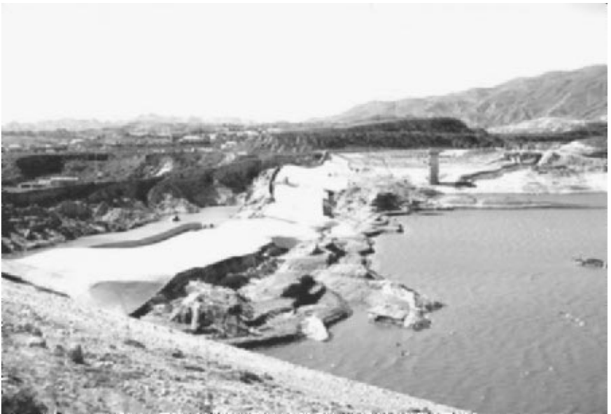
FIGURE 3.40 Flow slide of the Lower San Fernando Dam caused by the San Fernando earthquake on February 9, 1971. The photograph is a view to the west and shows the dam failure after the reservoir has been partly emptied. (Photograph from the Steinbrugge Collection, EERC, University of California, Berkeley.)
