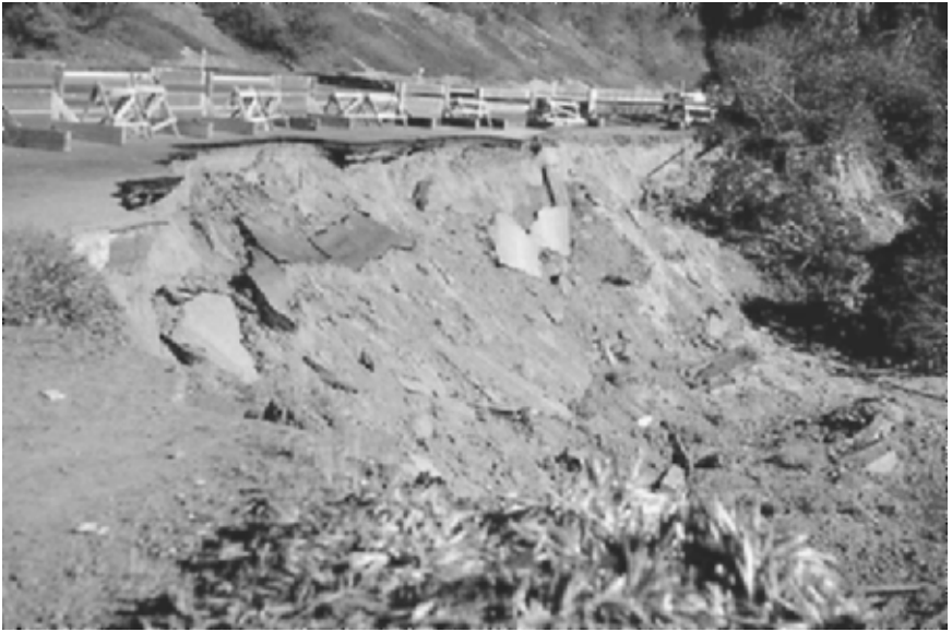
FIGURE 9.36 One of several earthquake-induced slides along Skyline Boulevard at Lake Merced, San Francisco. The slides were caused by the Daly City earthquake in California on March 22, 1957. (Photograph from the Steinbrugge Collection, EERC, University of California, Berkeley.)
