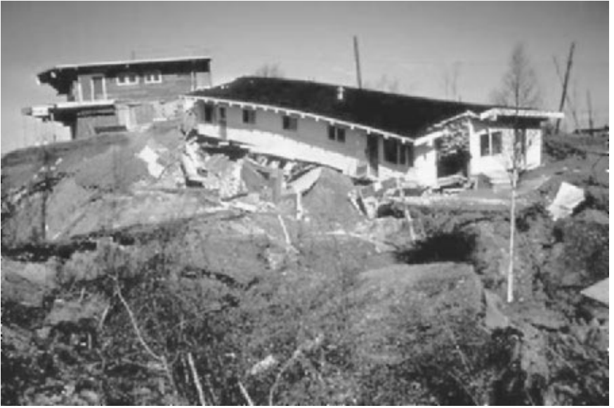
FIGURE 3.47 Damage caused by movement of the Turnagain Heights landslide during the Prince William Sound earthquake in Alaska on March 27, 1964. (Photograph from the Godden Collection, EERC, University of California, Berkeley.)
