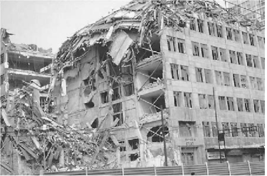
FIGURE 4.23 Building collapse in Mexico City caused by the Michoacan earthquake in Mexico on September 19, 1985. (Photograph from the Steinbrugge Collection, EERC, University of California, Berkeley.)
