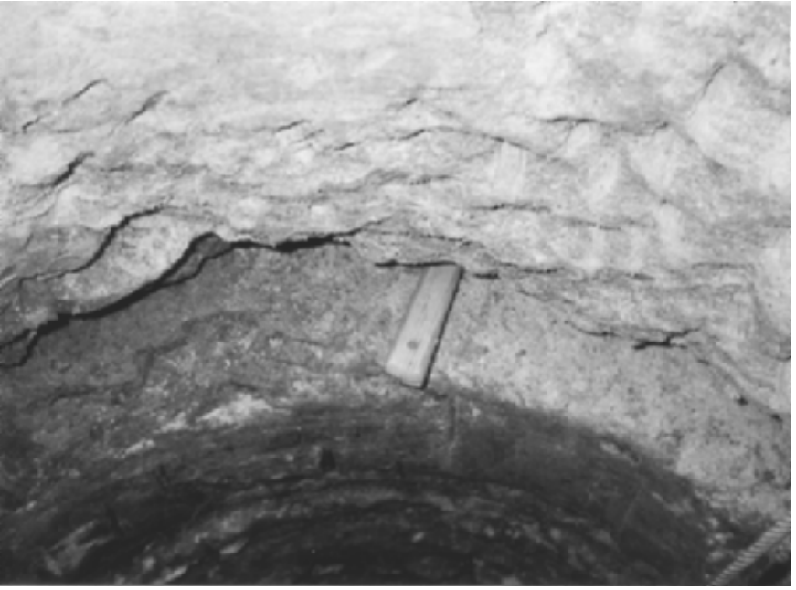
FIGURE 5.6 Knife placed in an open fracture in bedrock caused by landslide movement. The photograph was taken down-hole in a large-diameter auger boring.
