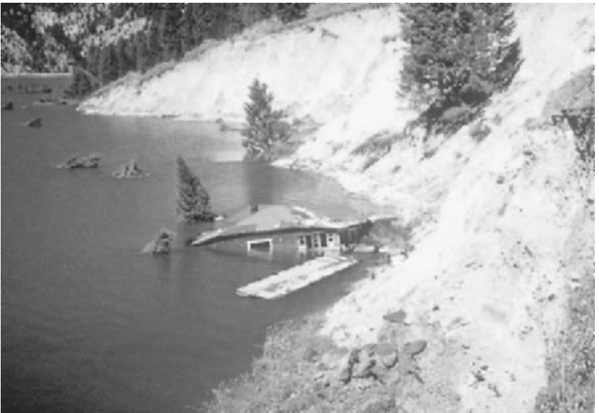
FIGURE 3.59 The building in the water was formerly on the shore about one-quarter mile up the lake. The house was apparently jarred from its foundation by the earthquake and then washed into the lake by the seiche generated during the Hebgen Lake earthquake in Montana on August 17, 1959. The house later drifted into the earthquake-created harbor shown in the above photograph. (Photograph from the Steinbrugge Collection, EERC, University of California, Berkeley.)
