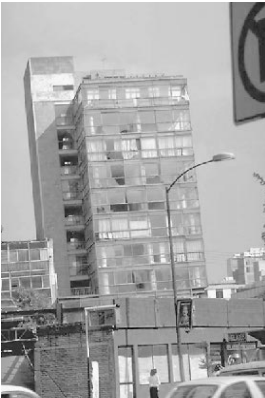
FIGURE 4.25 Building damage and tilting in Mexico City caused by the Michoacan earthquake in Mexico on September 19, 1985. (Photograph from the Steinbrugge Collection, EERC, University of California, Berkeley.)
