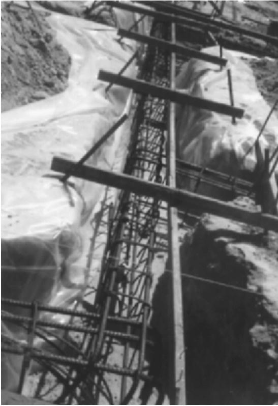
FIGURE 13.34 Overview of the steel reinforcement positioned within the grade beam excavation.
