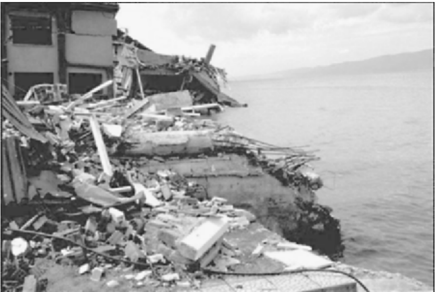
FIGURE 3.17 Flooding caused by regional subsidence associated with the Izmit (Turkey) earthquake on August 17, 1999. (Photograph from the Izmit Collection, EERC, University of California, Berkeley.)
