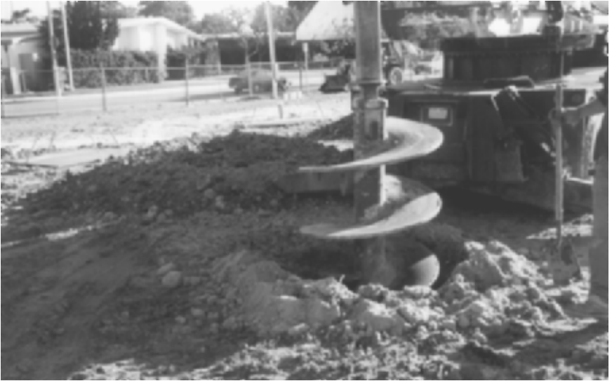
FIGURE 13.7 Close-up of auger being pushed into the soil.
