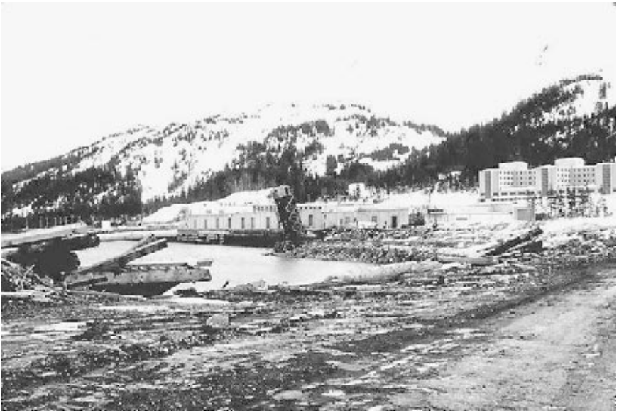
FIGURE 4.1 Overview of damage caused by a tsunami generated during the Prince William Sound earthquake in Alaska on March 27, 1964. Note the tilted tower in the background. (Photograph from the Steinbrugge Collection, EERC, University of California, Berkeley.)
