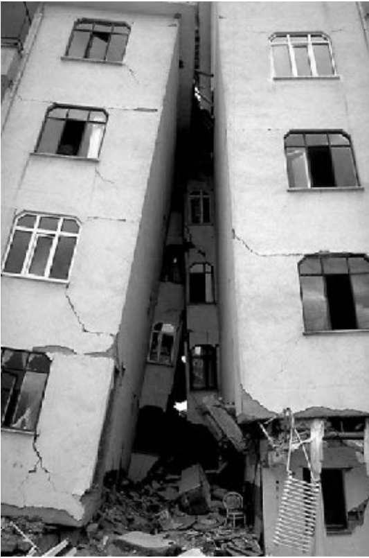
FIGURE 4.21 Another example of pounding damage and eventual collapse caused by the Izmit earthquake in Turkey on August 17, 1999. (Photograph from the Izmit Collection, EERC, University of California, Berkeley.)
