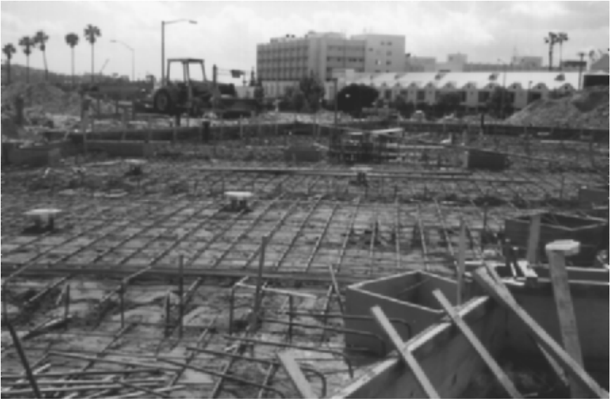
FIGURE 13.15 Positioning of the steel reinforcement for the floor slab.
