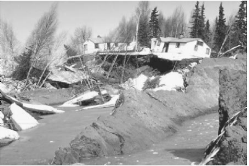
FIGURE 3.51 Damage caused by movement of the Turnagain Heights landslide during the Prince William Sound earthquake in Alaska on March 27, 1964. (Photograph from the Steinbrugge Collection, EERC, University of California, Berkeley.)
