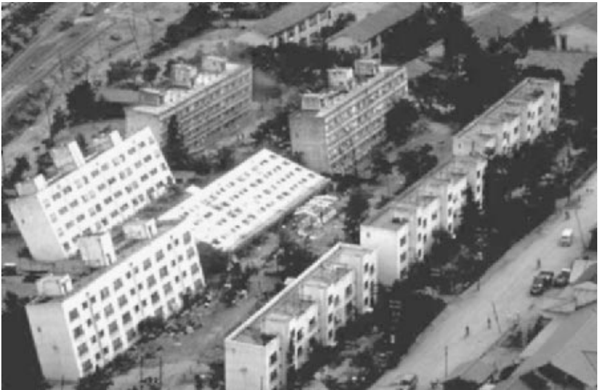
FIGURE 3.20 Kawagishi-cho apartment buildings located in Niigata, Japan. The buildings suffered liquefaction-induced bearing capacity failures during the Niigata earthquake on June 16, 1964. (Photograph from the Godden Collection, EERC, University of California, Berkeley.)
