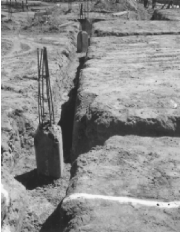
FIGURE 13.29 Prestressed concrete piles have been installed, and the excavations for the pile caps and grade beams are complete. The strands at the top of the pile will be connected to the steel reinforcement in the pile cap and grade beam.
