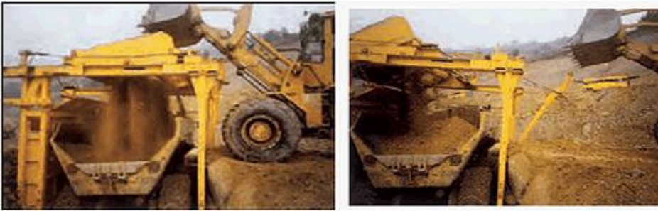
Criblage (source SETRA)
