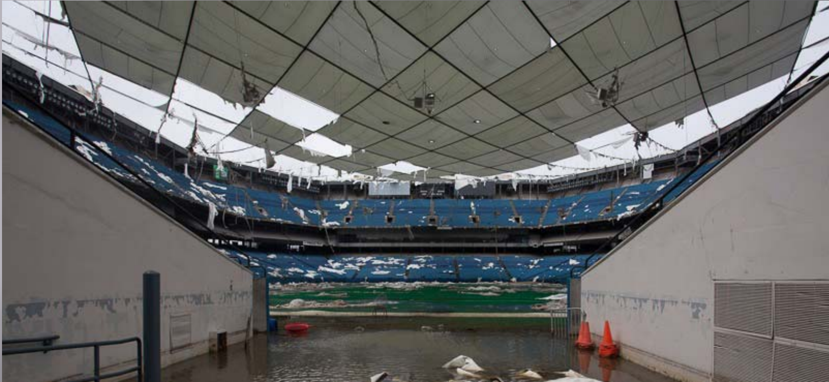
Pontiac Silverdome (U.S.A) Air-Inflated Structure (Pneumatic Structure)
