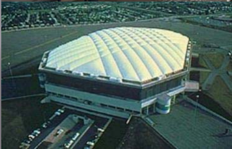
Pontiac Silverdome (U.S.A) Air-Inflated Structure (Pneumatic Structure)
