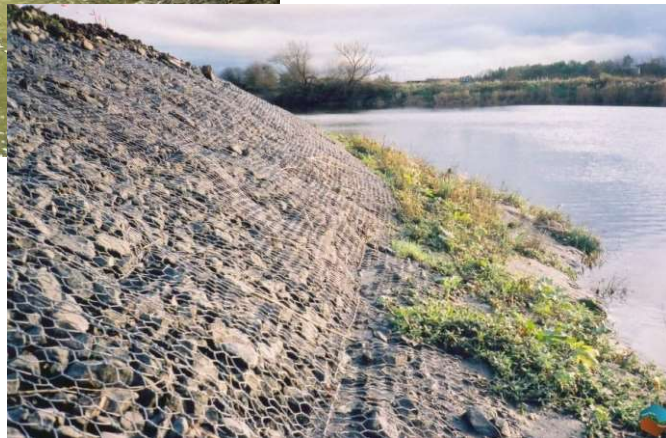
Matelas-gabions et gabions
