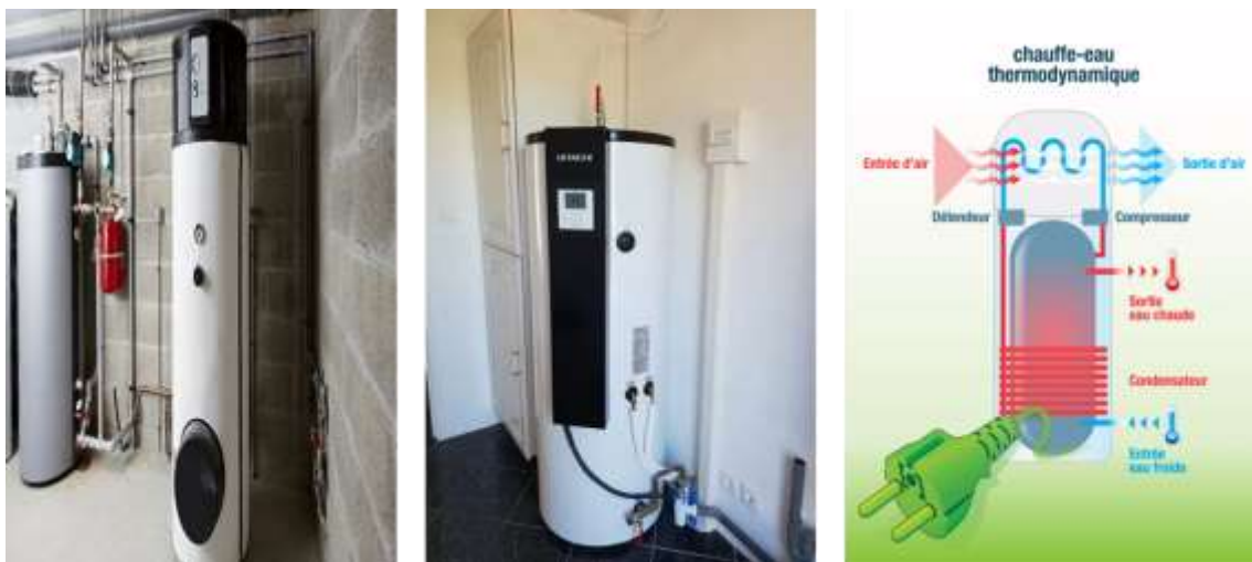
Figure III.5 : Chauffe-eau thermodynamique
